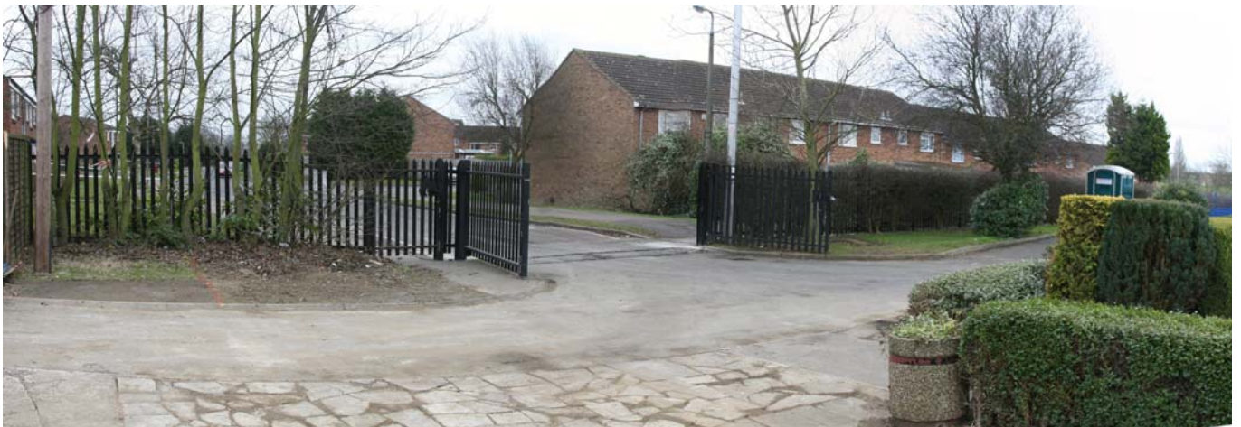
Image 02: Existing Main Vehicular and Pedestrian Gates
