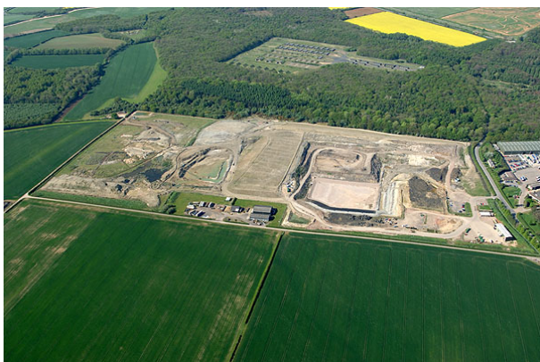
The East Northants Resource Management Facility
