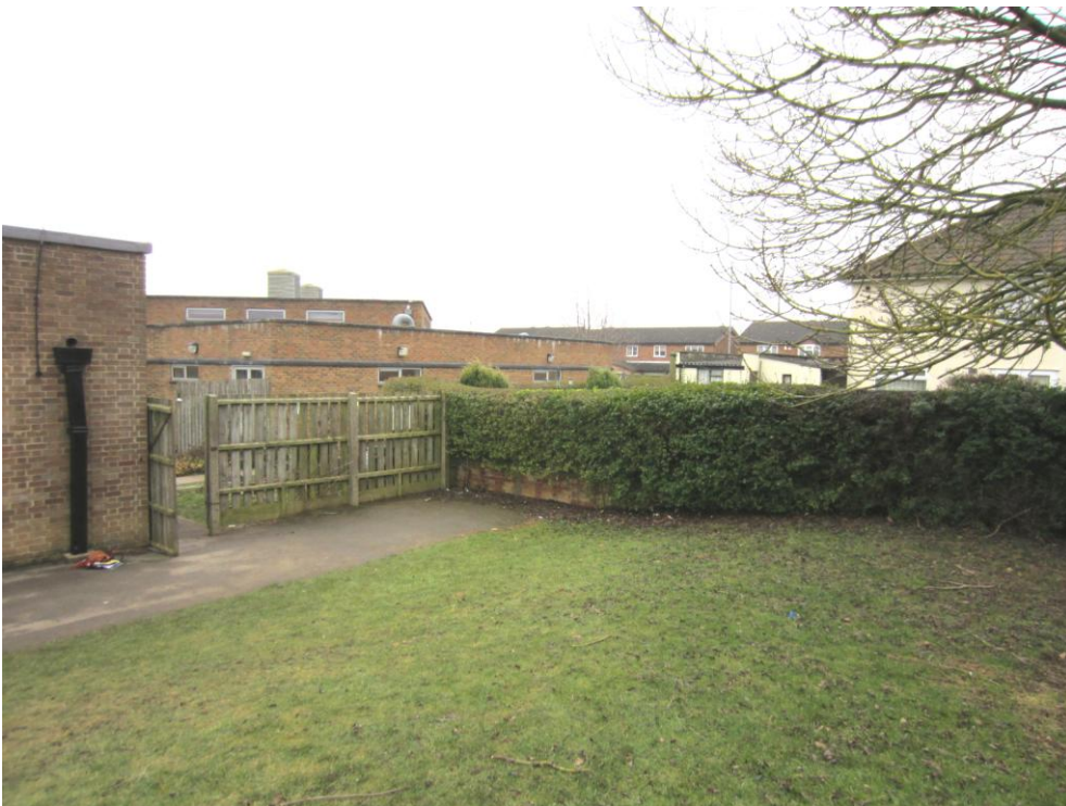
Gates and fence in southeast corner of site
