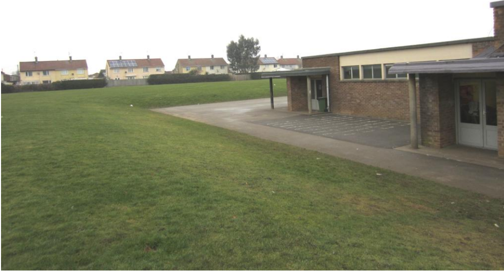
Proposed site from the south with access doors into main building
