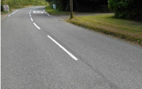
It extends the life of the road surface, increases skid resistance and seals the surface to stop water ingress, protecting it from damage caused by severe winter weather, such as potholes.
